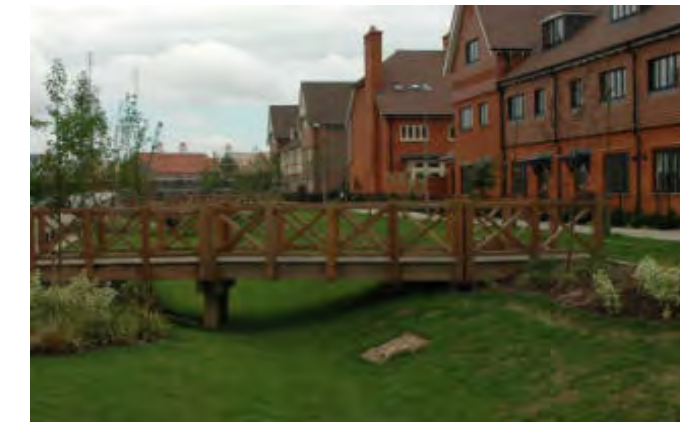
Simple dry swale running along street
