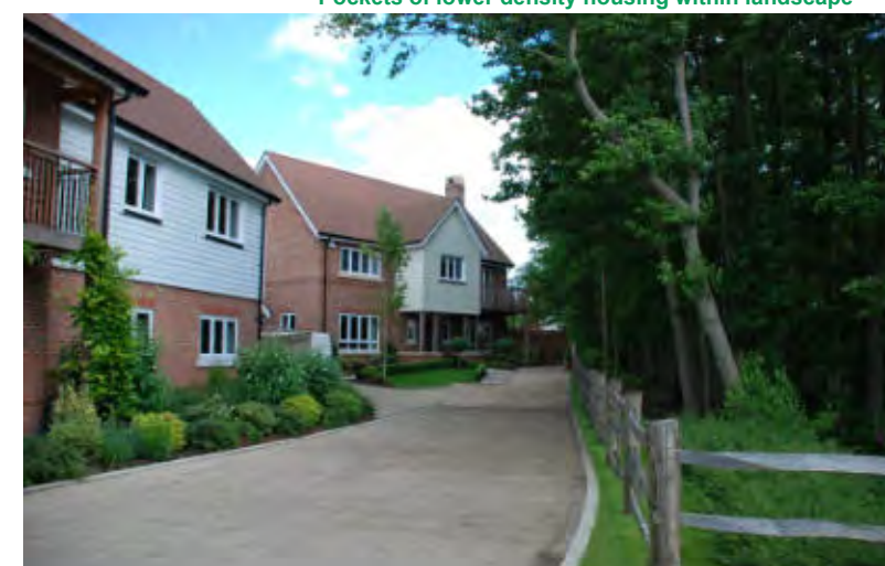
Larger properties which front on to open space with access lanes
