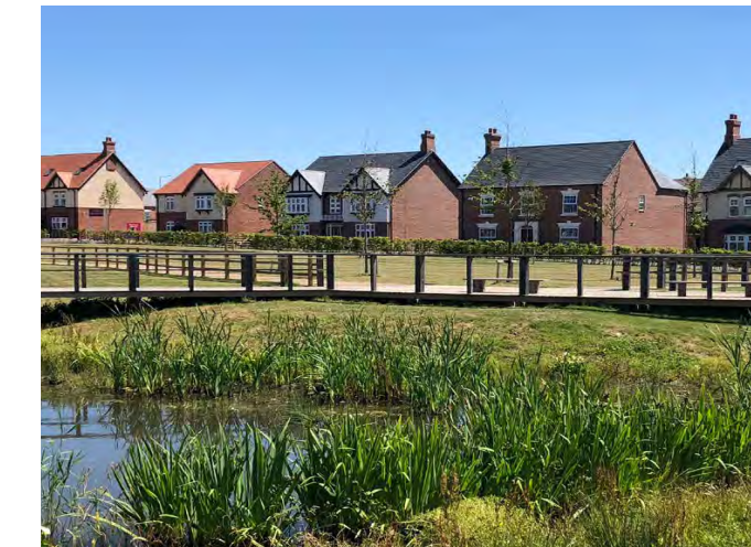
SuDS basin integrated into green corridor
