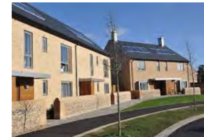
RENEWABLE ENERGY TECHNOLOGY CAREFULLY CONSIDERED IN STREETScape
